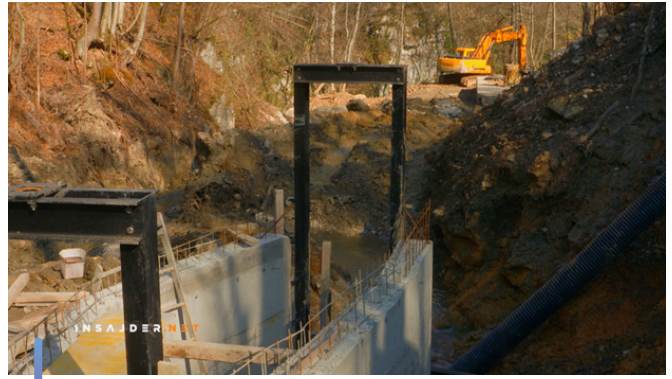
Construction works on the SHPP “Jovanovići”, source: Insider, November 2018: https://insajder.net/sr/sajt/tema/12529/
